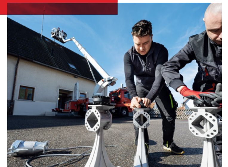
> Installation team for the HÖRMANN sirens
